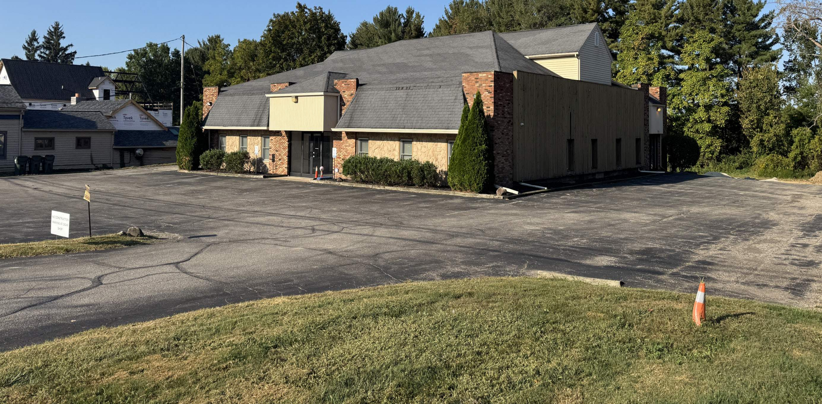
Existing North East Corner
