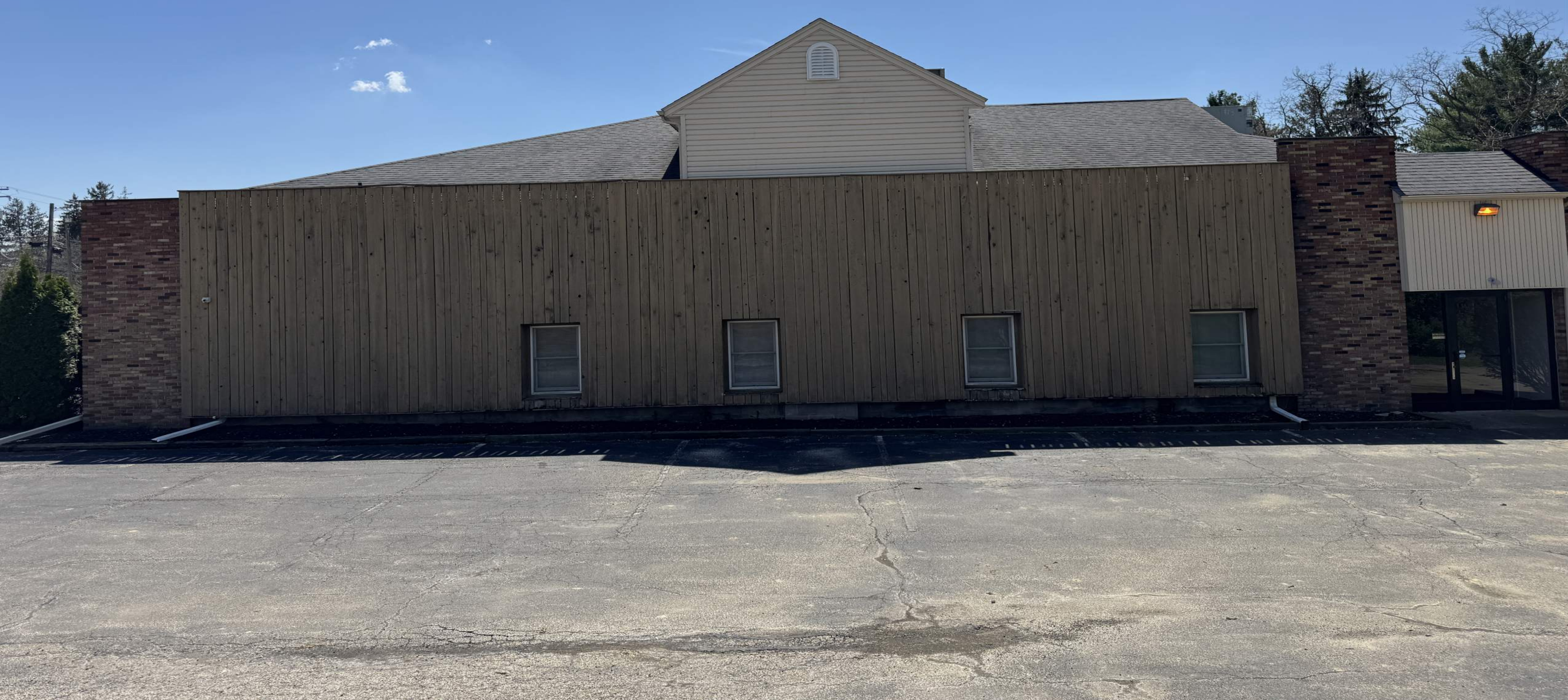
Existing North Side
