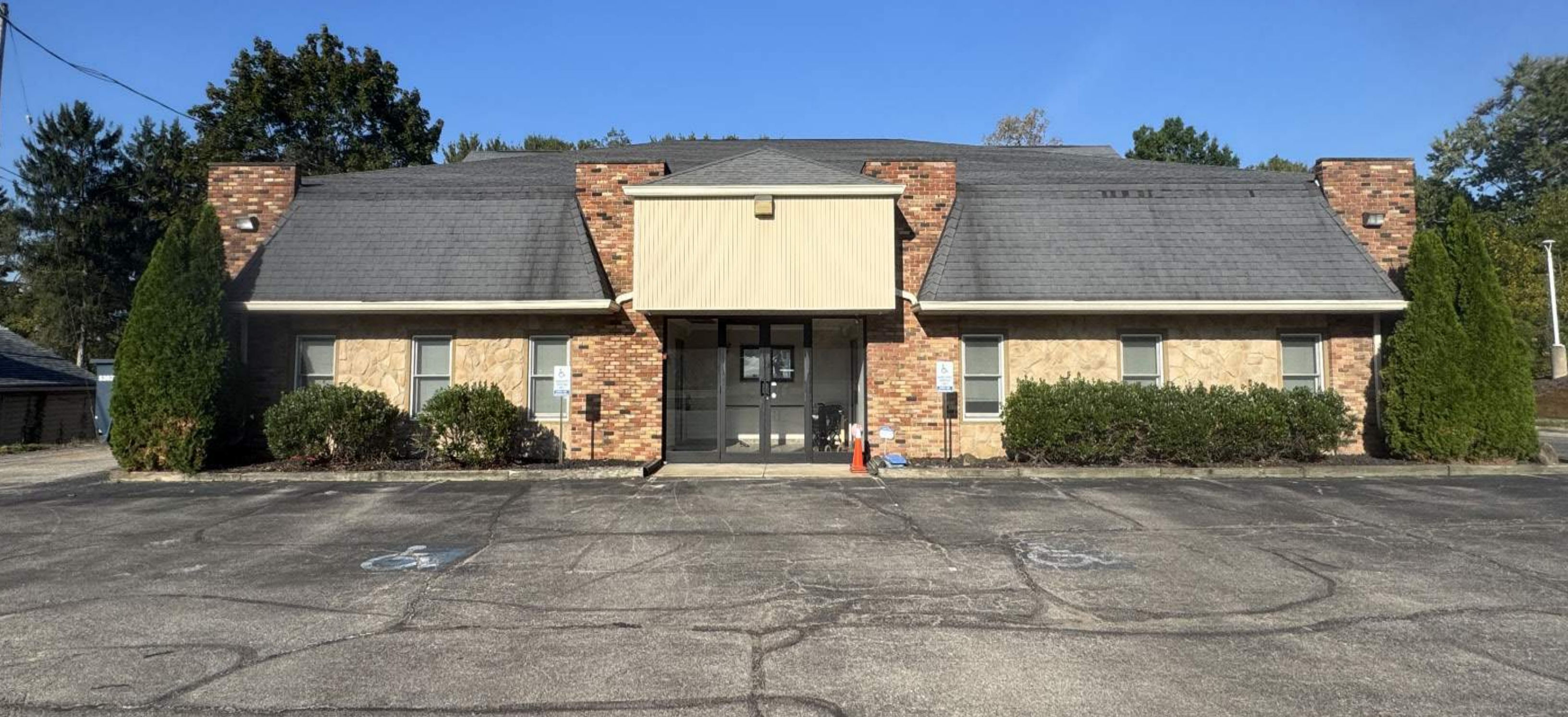
Existing Front Entry
