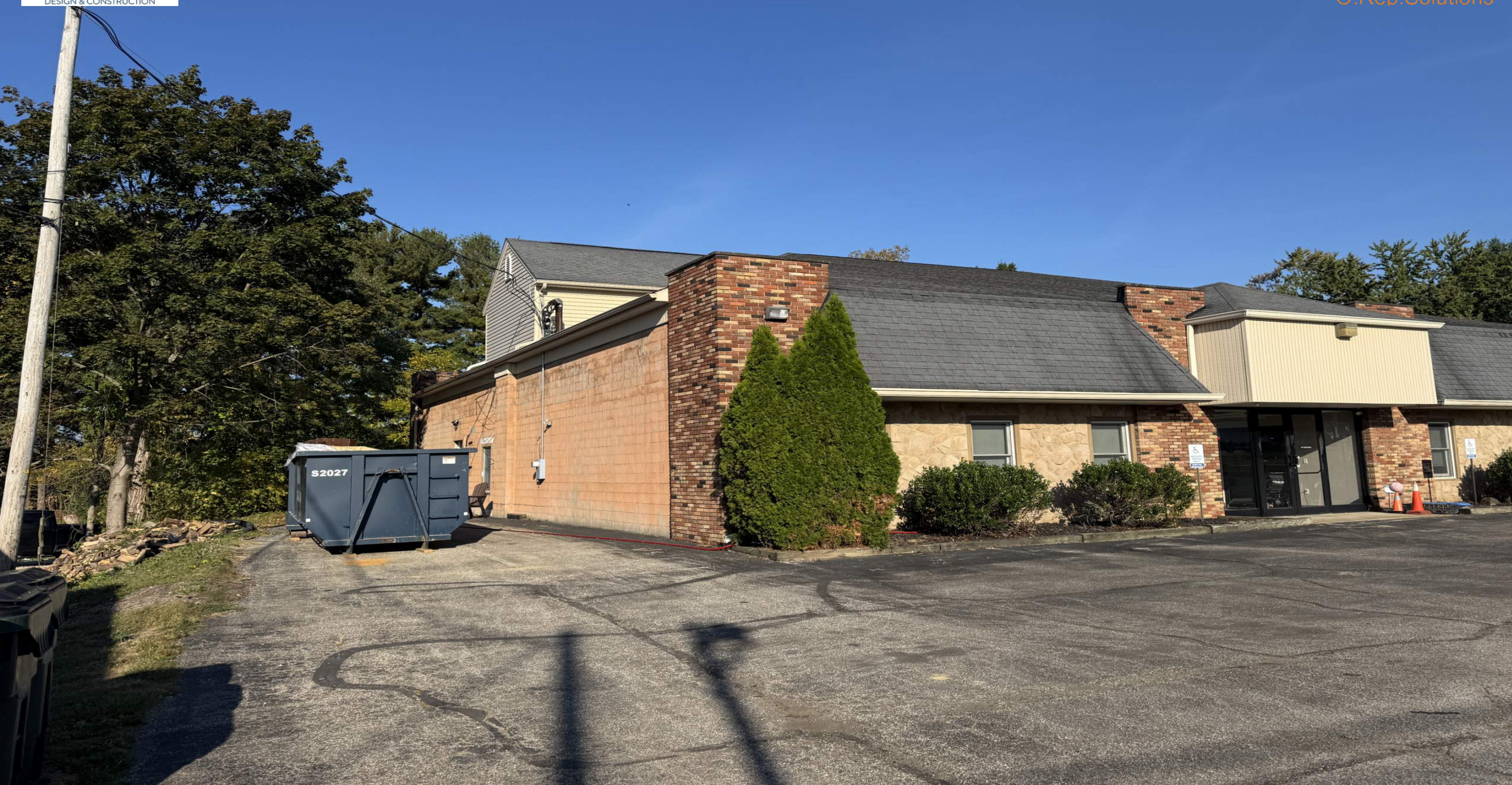
Existing South East Corner
