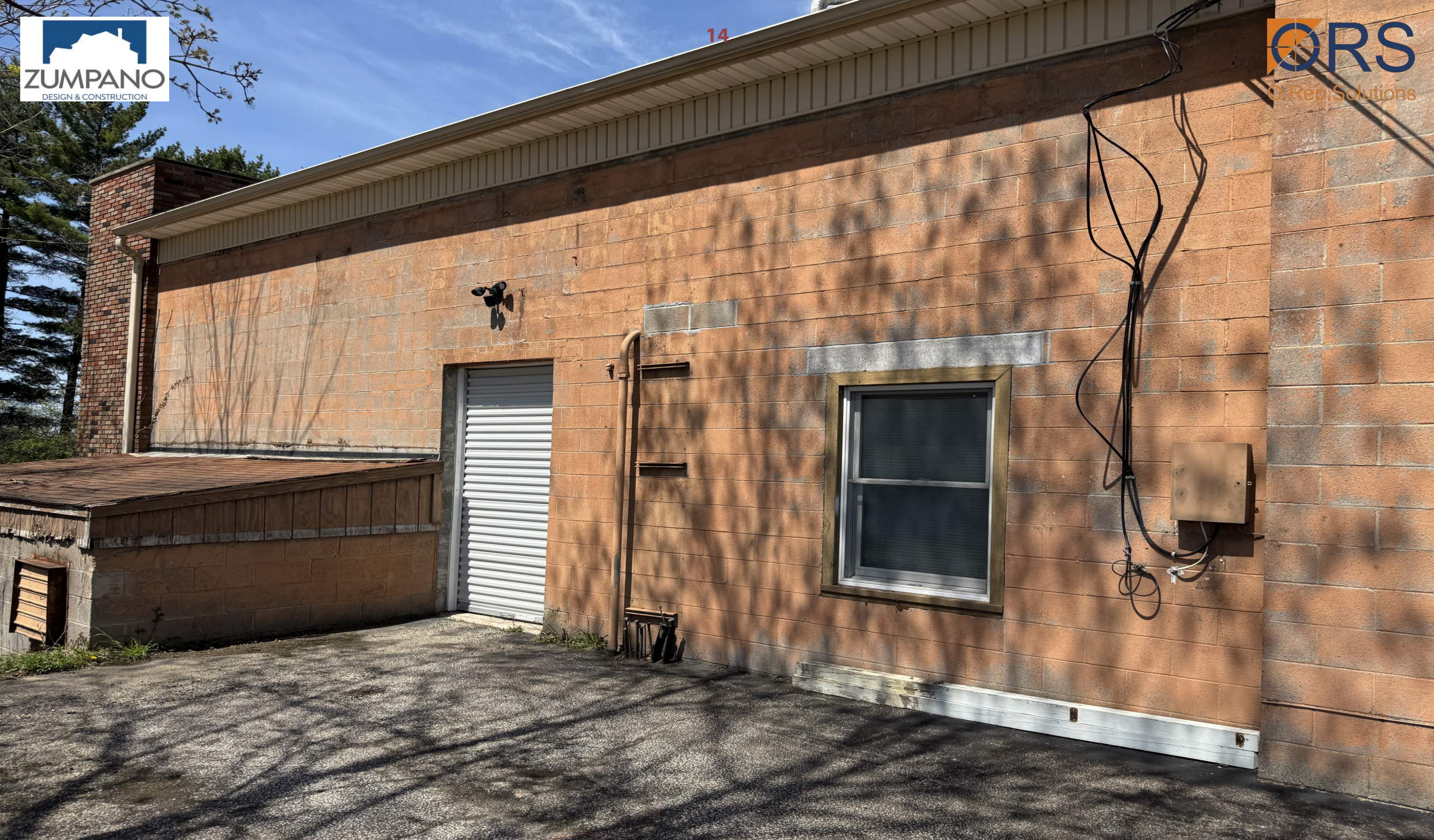
Existing South Side
